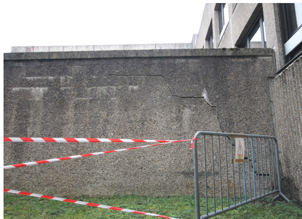
Fissure structurelle
